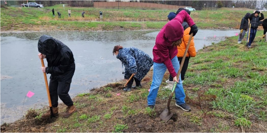
Figure 7. SES students dig holes to plant dogwood and osier trees around a bioretention basin and iron-enhanced sand filter project in Lakeville in April 2023.
